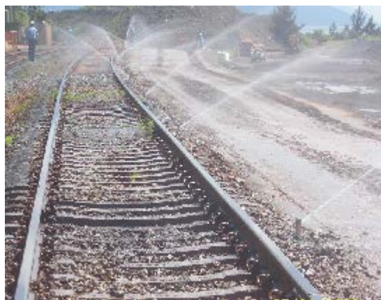
Figure 5-4: Water sprays along the loading/unloading points
