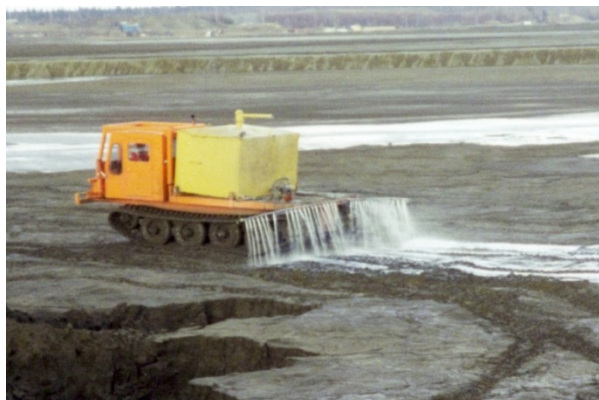
Figure 5-12: Dust suppressant application on tailings
