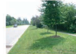
Limiting road width to a minimum allows the remainder of the ROW to act as a buffer
