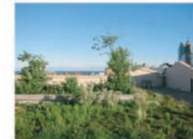
Rooftop gardens lower the local temperature, retain water and can provide amenity space.
