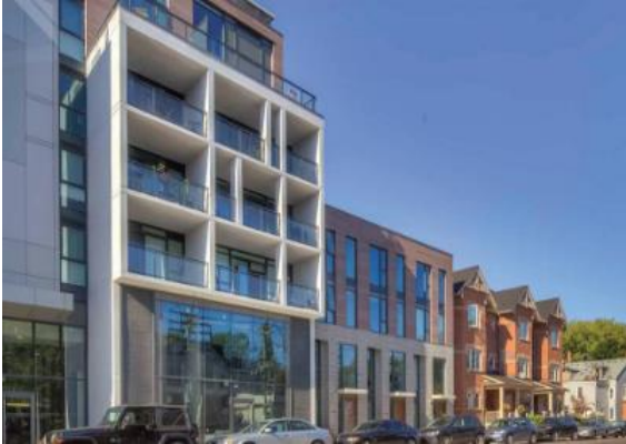
Transition in building forms from mid-rise to low-rise buildings
