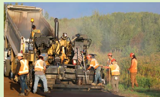
Figure 3. FPIinnovations – Lignin Modified Asphalt Test Sections
